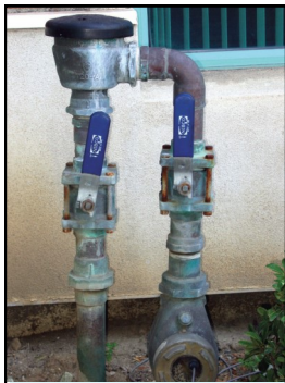
Pressure Vacuum Breaker (PVB)
